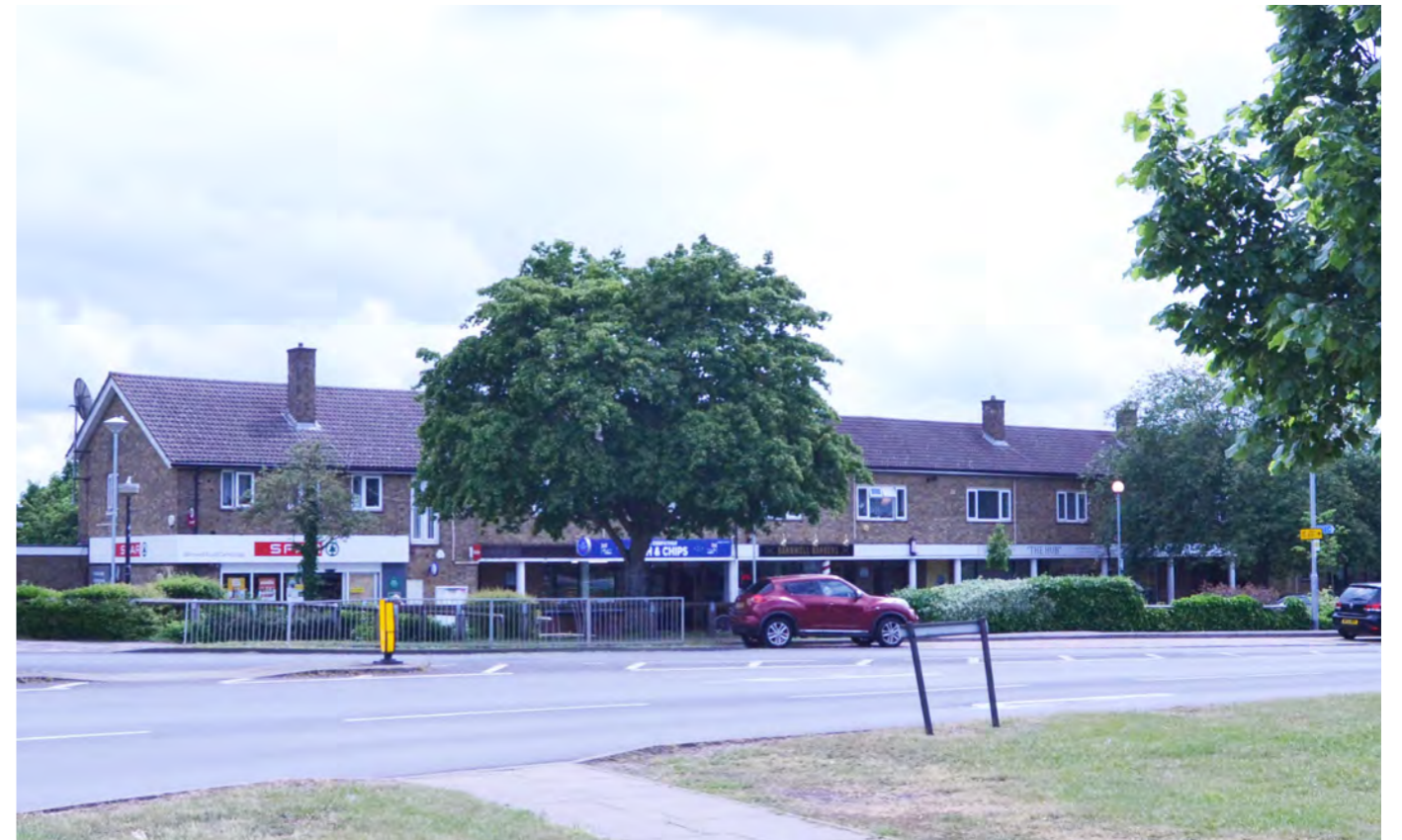
Site 2 - View of existing shops
